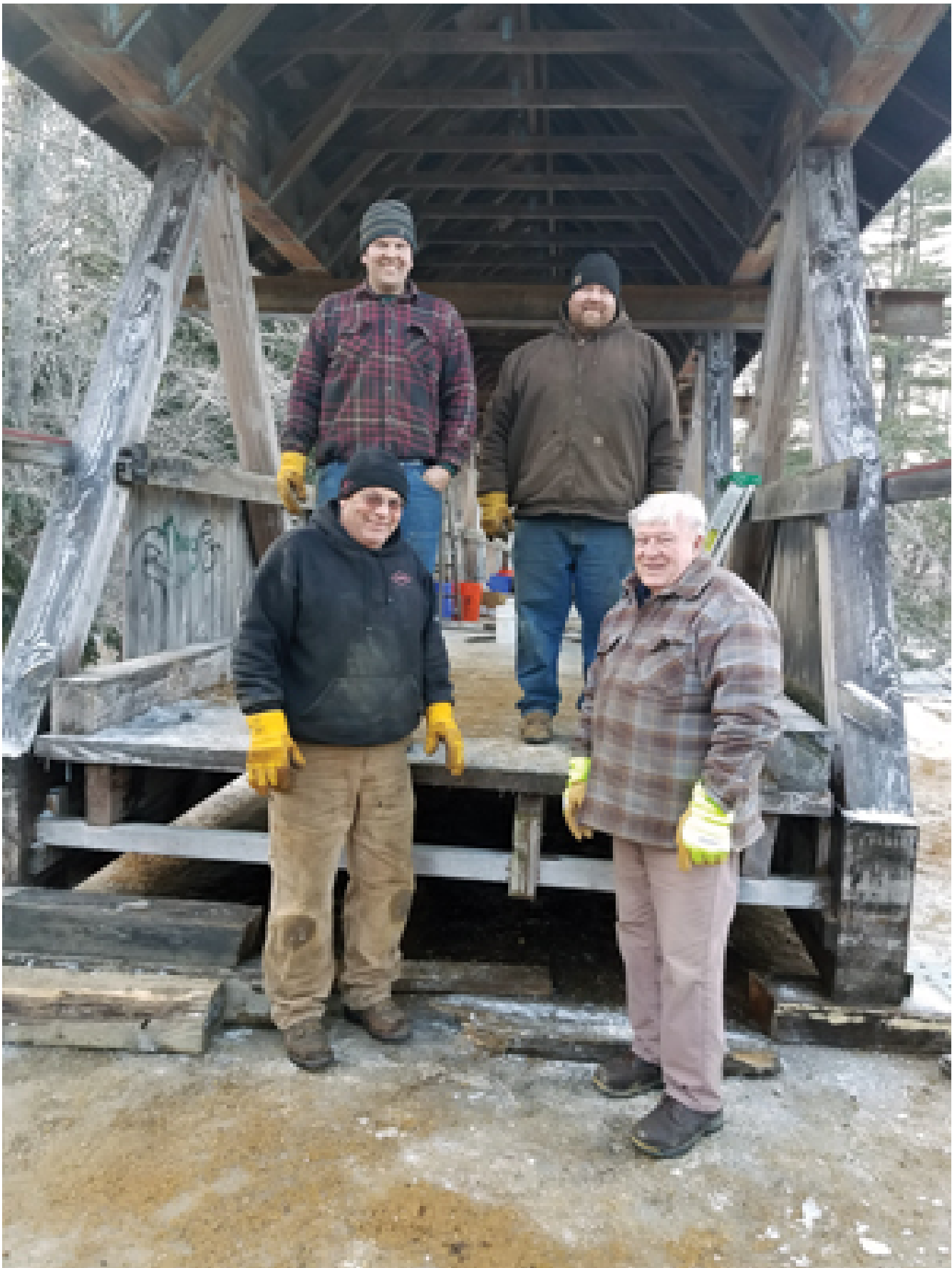
Mark, Matt and Jeff Roberts, along with Ron Mitchell, were among the volunteers who installed the old bridge in Belmont recently. (Courtesy photo)
